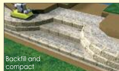
Install wall out from stairs
