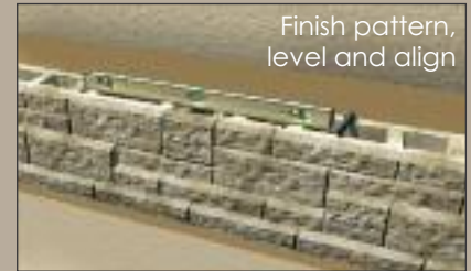
Compact on block and behind
