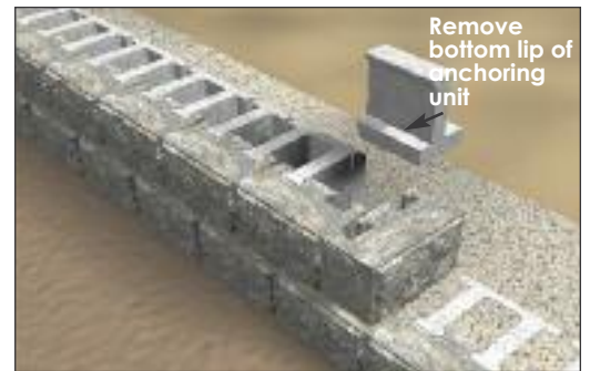
Modify half an anchoring unit by removing lip to secure the facing unit.
